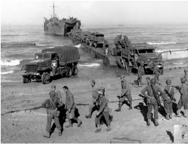
LST Discharging Cargo over a Pontoon Causeway
