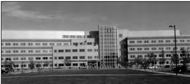
Figure 1. TRADOC Headquarters, Fort Eustis, Virginia.
